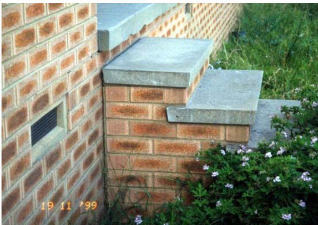
Figure 3a - Stepped brick crack at south-west corner below DPC
