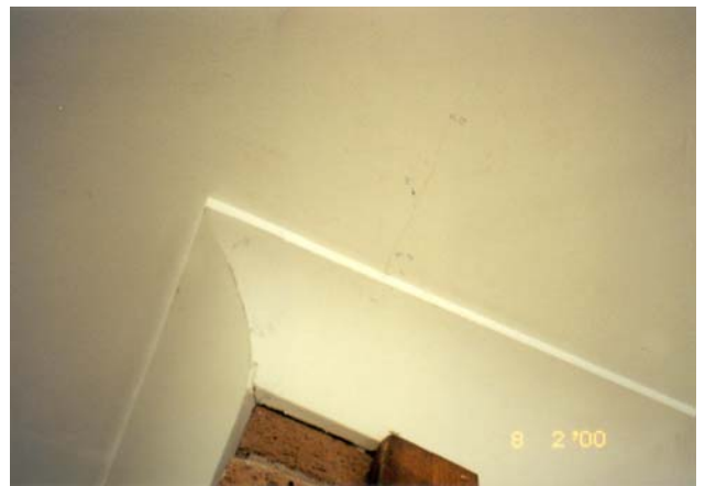
Figure 3l - Shrinkage crack in concrete verandah slab
