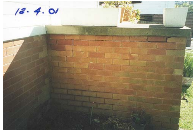
Figure 29n – Reference House R6 (Kotara) – rotated corner
