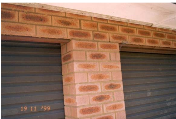
Figure 3g - Freestanding wall moves independently of the garage
