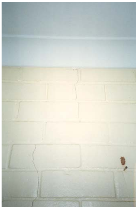
Figure 3m - Inclined plaster crack in kitchen from window to encased beam
