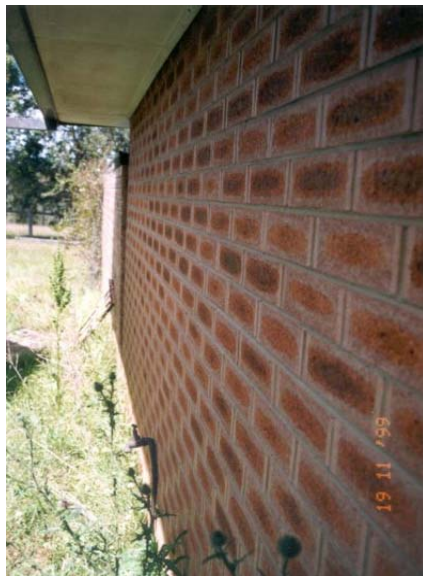
Figure 3e - Horizontal mortar crack between toilet and bathroom windows
