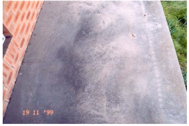
Figure 3l - Shrinkage crack in concrete verandah slab
