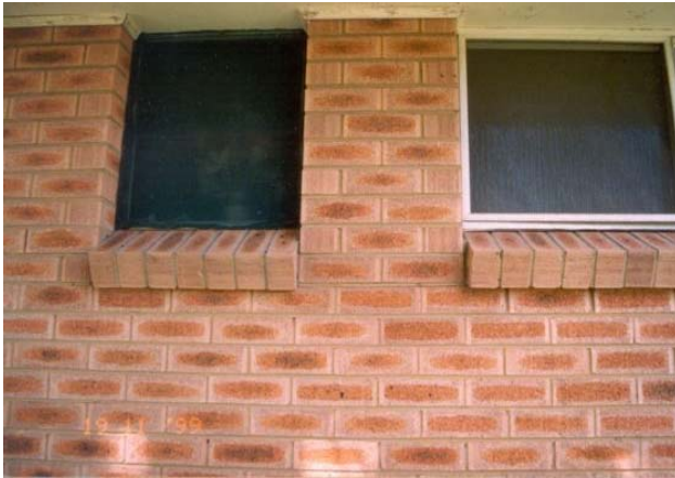
Figure 3e - Horizontal mortar crack between toilet and bathroom windows
