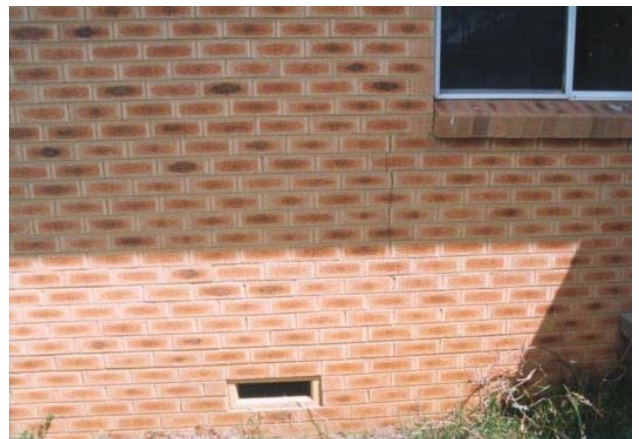
Figure 3b - Stepped brick cracks below DPC at south-west corner
