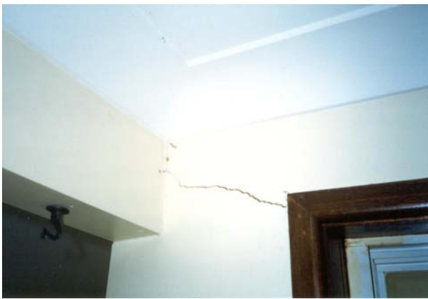
Figure 3m - Inclined plaster crack in kitchen from window to encased beam
