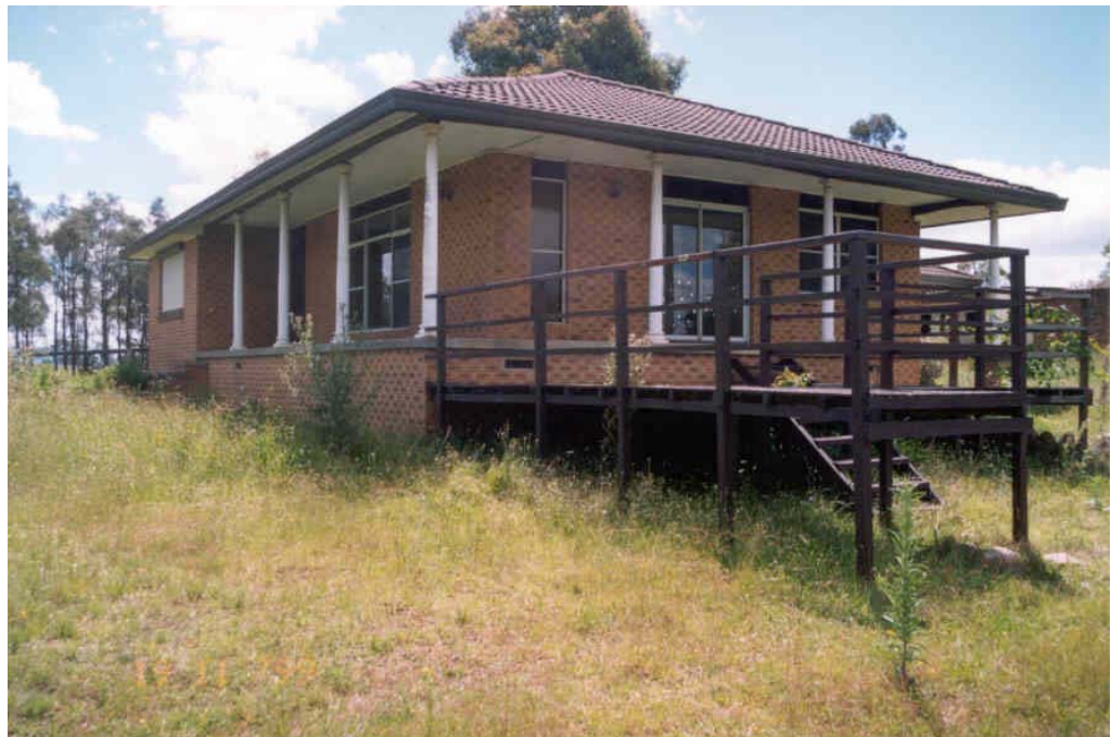
Figure 2 – South-east view of Rix's Creek test house
