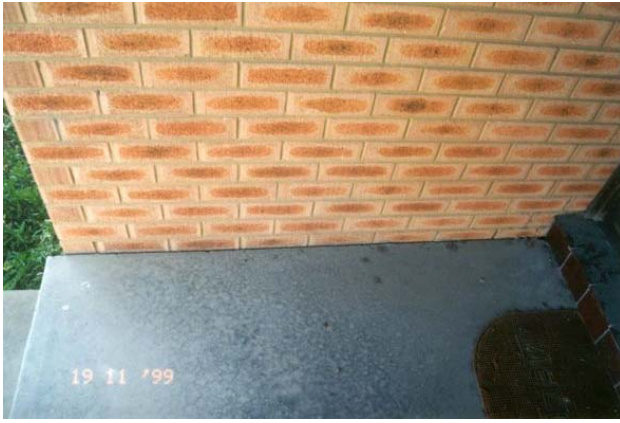
Figure 3k - Separation of path from wall
